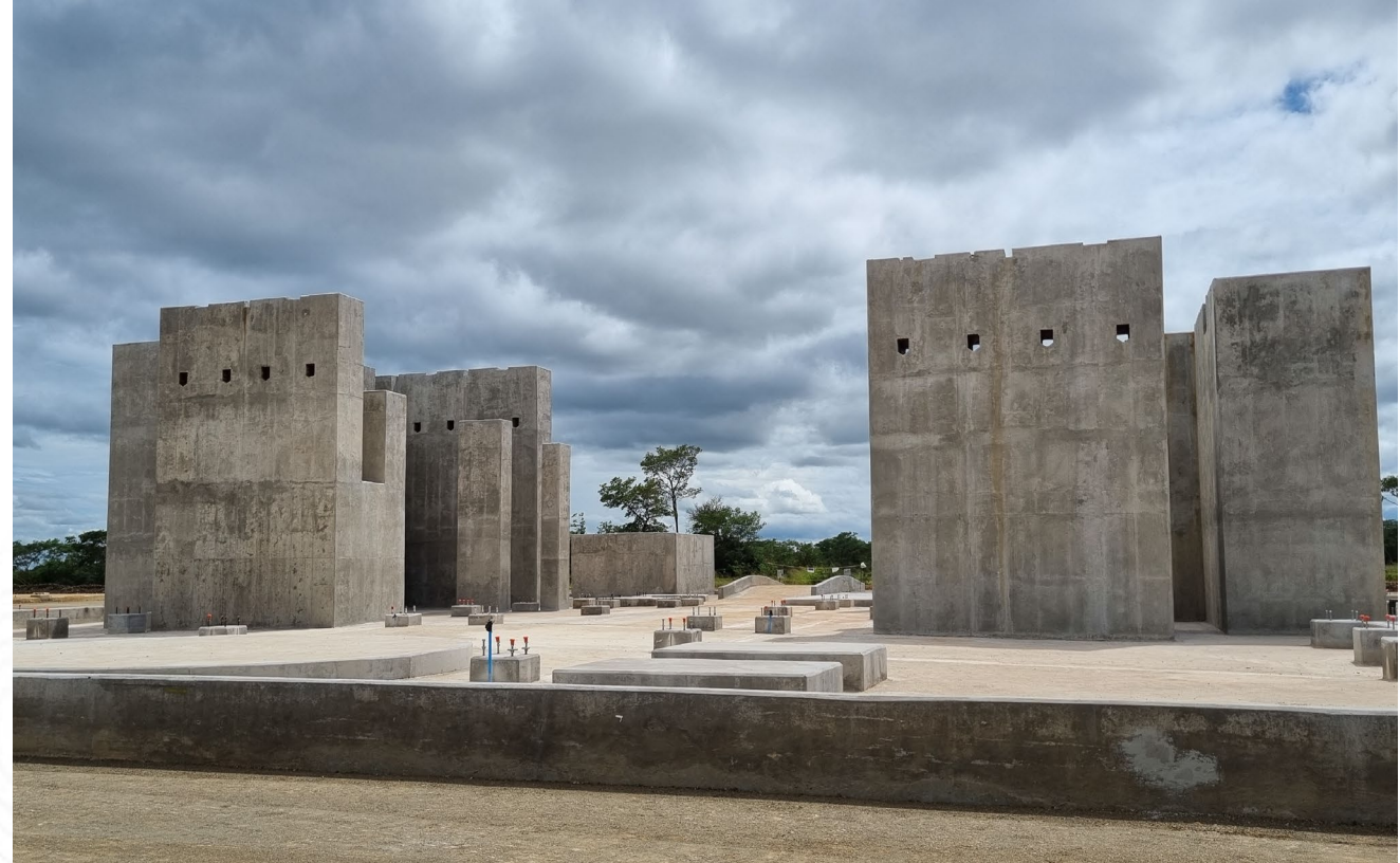
Primary and secondary mill foundations - completed
