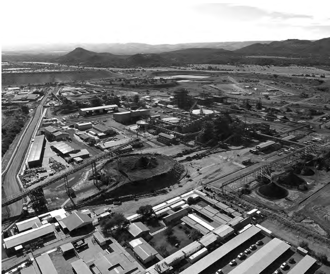
Tharisa processing facilities with Voyager Plant in the foreground
